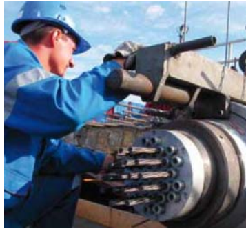
Figure 3.6 – Hydraulic jacking of wedge anchorage (Freyssinet, 2010a)
